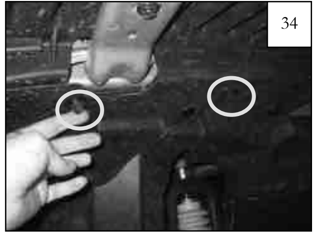
Reinstall two factory bolts as shown as well as reinstall marker light wiring.
