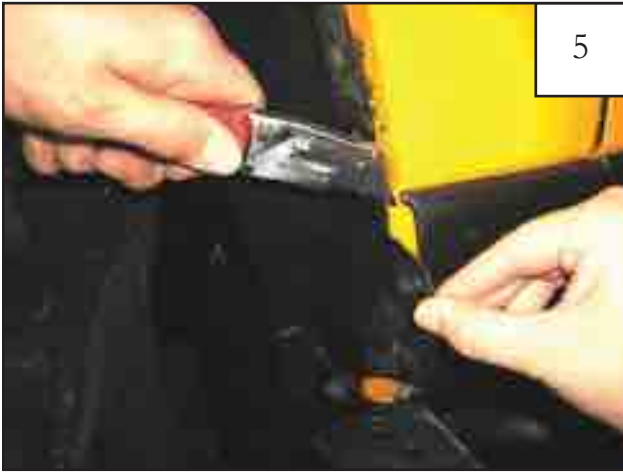
Using a utility knife, cut splash guard flush with edge of a sheet metal.
