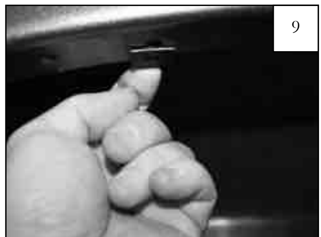
Install Clip (CL1-0022) over existing hole.
