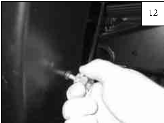
Using #2 Phillips Screwdriver, insert a supplied Screw (SW1-0056) through existing holes in flare and into holes in clips (4 places).
